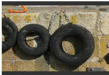
Gambar 7.4: Fender Ban Bekas Mobil
